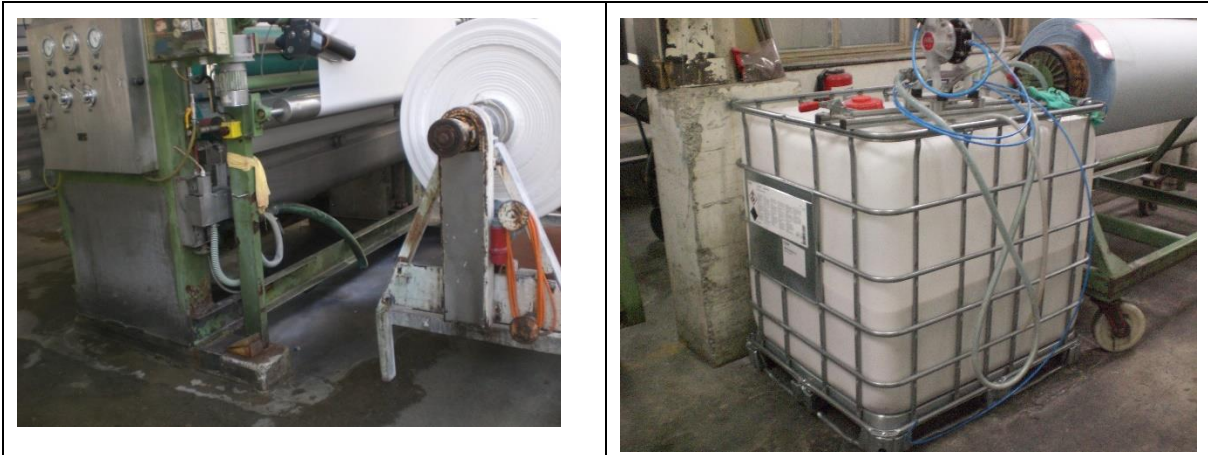
Figure 7: On the left, the photo shows the padder of a stenter and on the right an intermediate bulk container (IBC) equipped with a pump and pipes to manually empty the padder (Photos: Dr. Harald Schönberger)
